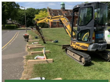
Installation of hundreds of posts by Brentwood Council
